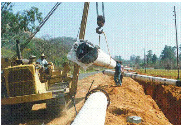
Figure 14: Trench and working area for pipe lying
